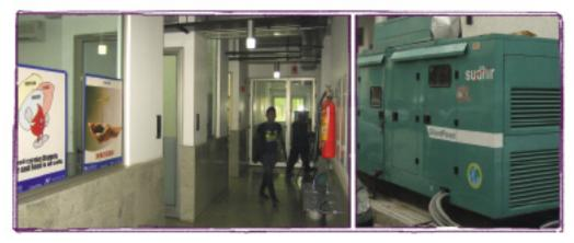
A 320 kVA-generator now secures the electricity supply for cooling blood bottles in case of power cuts in a blood preservation project in New Delhi.
