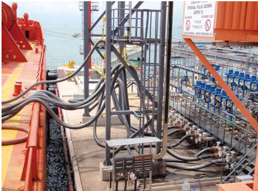
NEW LIFTING METHOD One of several advantages of the new marine jetty 10 in Singapore.
