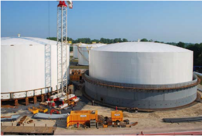
A SIDEWAYS MOVE OF SEVEN METERS was crucial to meet the necessary safety distances during the reconstruction of the Honau terminal. The tank was jacked up on wood and, with the help of nitrogen, shifted on rails.
