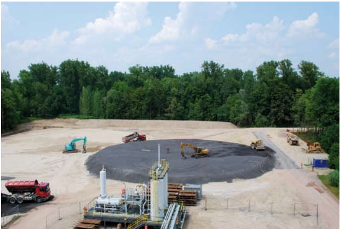
A SIDEWAYS MOVE OF SEVEN METERS was crucial to meet the necessary safety distances during the reconstruction of the Honau terminal. The tank was jacked up on wood and, with the help of nitrogen, shifted on rails.
