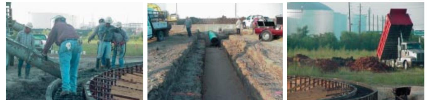
Building a new tank: Pouring and vibrating almost simultaneously.
