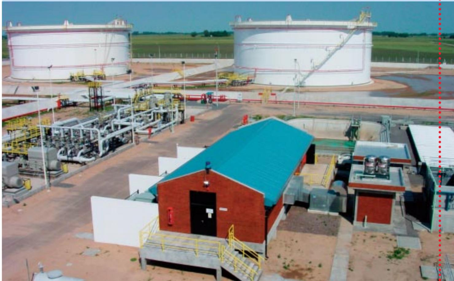
The new facility includes a new storage terminal with a total of 60,000 cbm of storage capacity, a complete pump station with a capacity of up to 20,000 cbm/day, and a 167 km long 22 inch diameter pipeline linking the new tank terminal with Esso's refinery in Campana.
