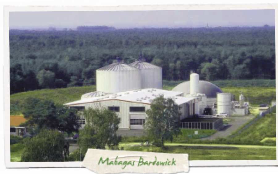
Mabagas took over an existing biogas plant in Bardowick near Lüneburg in 2012
